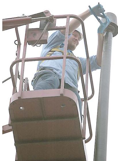
James Stanton adjusts the cable pulley device atop a 30-foot flagpole.
