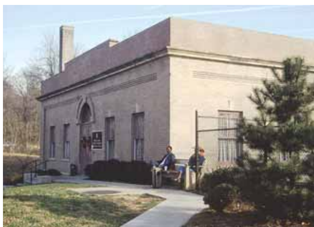
Exterior shot of Eleanor U. Kennedy Shelter located at 9155 Richmond Highway.
